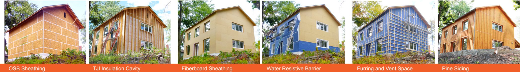
OSB Sheathing TJI Insulation Cavity Fiberboard Sheathing Water Resistive Barrier Furring and Vent Space Pine Siding
