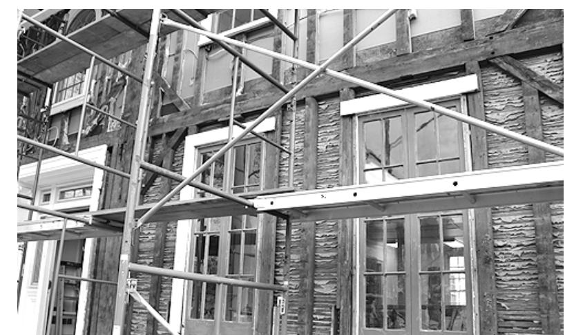
View of south wall restoration
